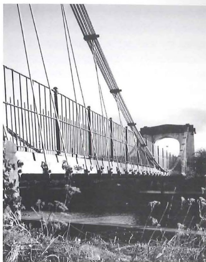
Fig.8 Victoria Bridge, an improved type of suspension bridge designed by James Dredge c.1837, to provide a crossing between the Upper and Lower Bristol Roads. (photograph James O. Davies)
